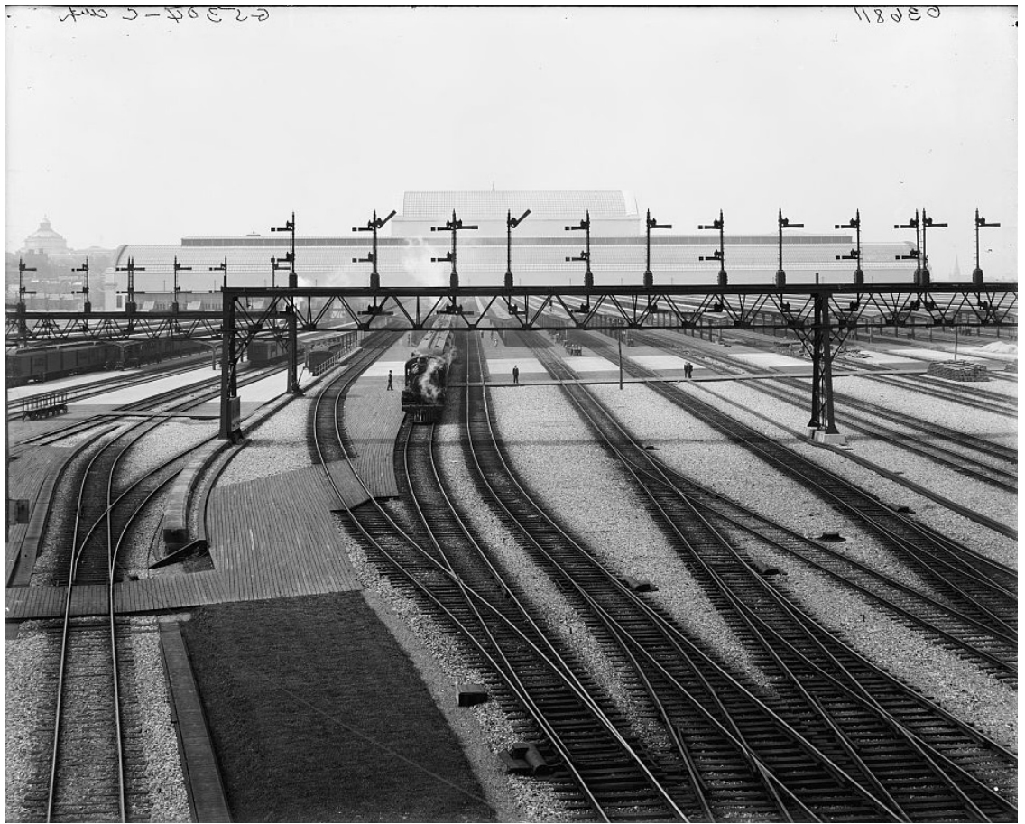
Right: Newly completed terminal throat and signals stretch out at Washington Union Station in 1907. Photograph courtesy of Library of Congress / Detroit Publishing Company
