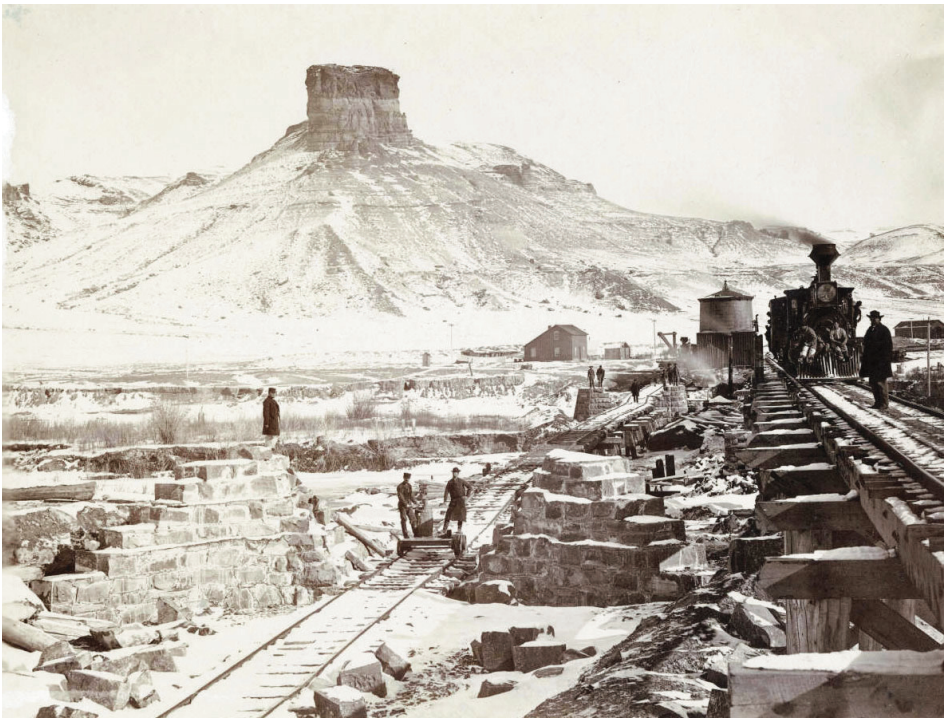
Left: Temporary and permanent bridges on the Union Pacific and Citadel Rock, Green River, Wyoming, 1868. Photograph by A.J. Russell and from Glenn Willumson's Iron Muse: Photographing the Transcontinental Railroad
