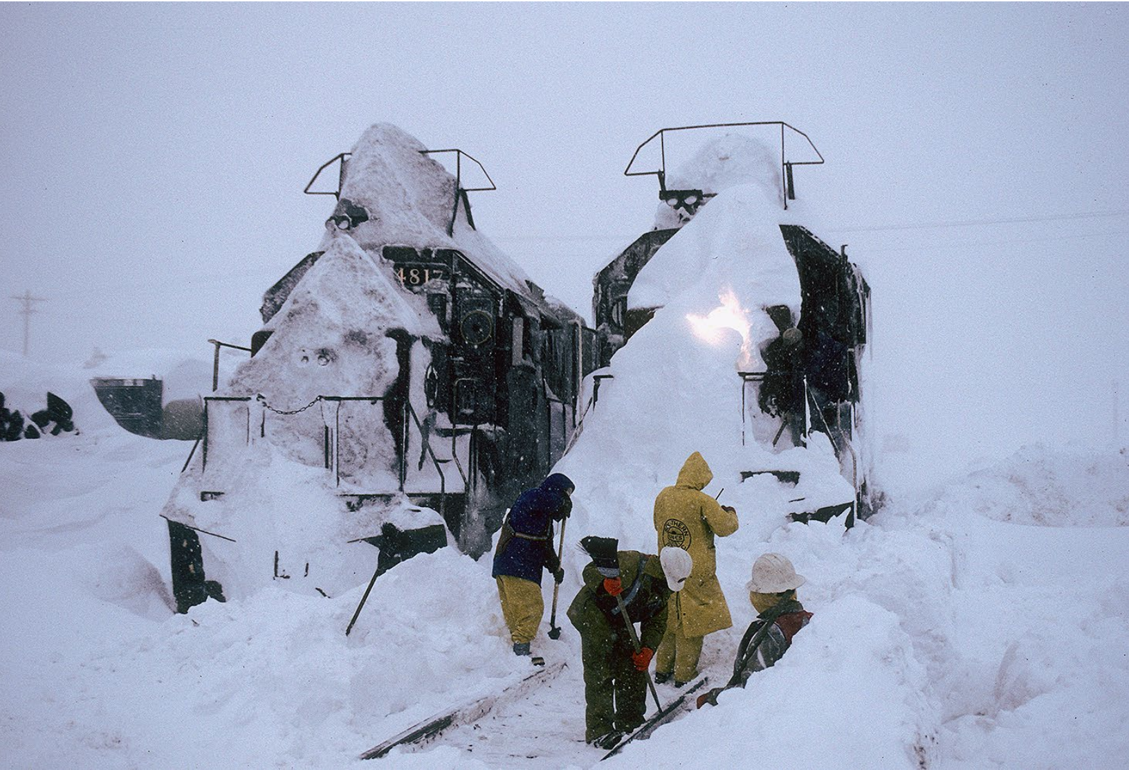
Union Pacific maintenance-of-way workers—still wearing Southern Pacific winter coats—dig snow out of a switch at Truckee, California, to get a flanger out for a trip west over Donner Pass on December 22, 1996. Photograph by Dick Dorn
