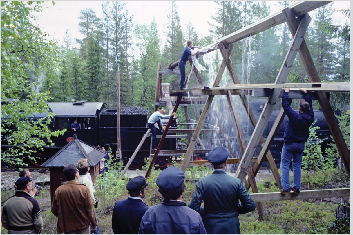
Right: Swedish State Railways workers demonstrate how to water the locomotives using a long wooden sluice that brings water through the forest to the tracks. Shot in July 1982, somewhere along the Inlandsbanan in the forested Swedish interior. Posner-23-06-18
