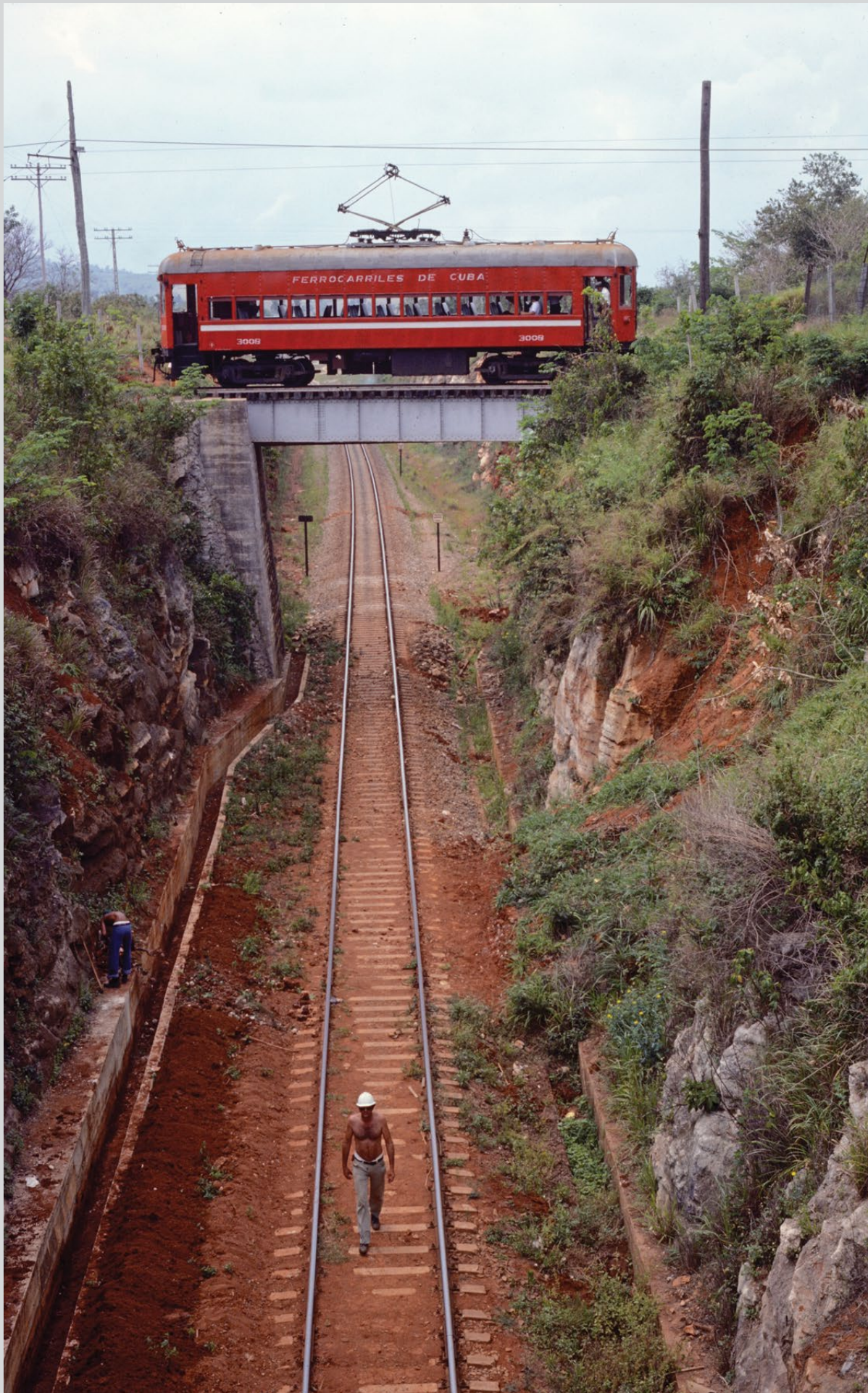
A one-car Ferrocarriles de Cuba electric passenger train crosses a bridge over a worker walking along another set of tracks on March 3, 1980. Posner-07-04-15
